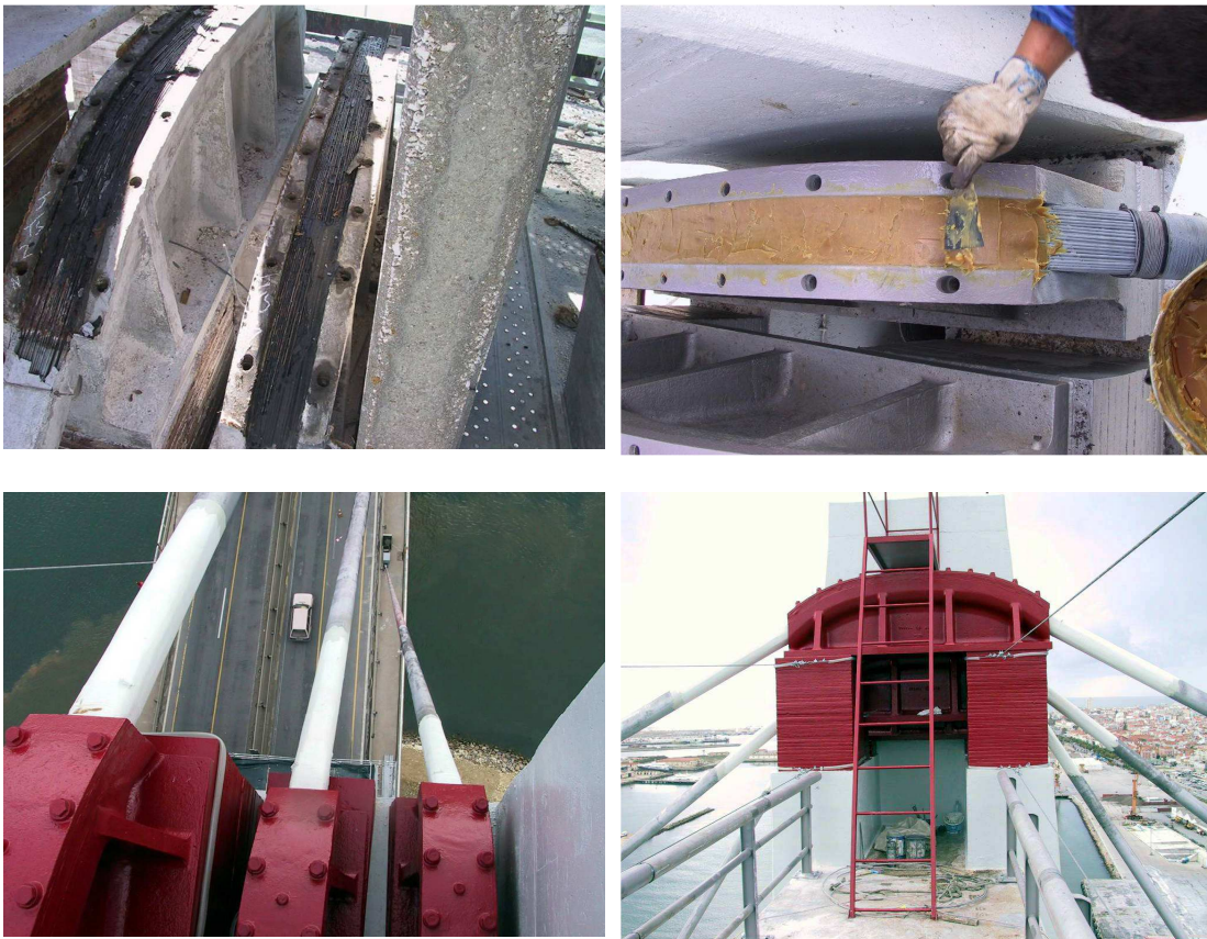
Figure 8. General rehabilitation of the saddles
