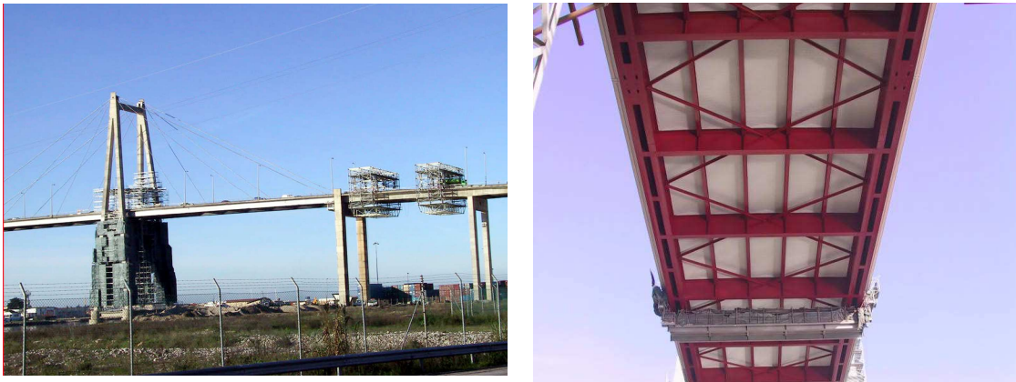
Figure 5. General view of the bridge under repair and working platforms
