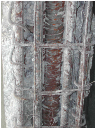
Repairing of the prestressed beams of the viaduct
