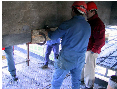
Repairing of the prestressed beams of the viaduct
