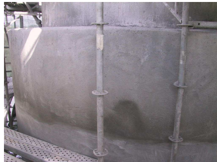
Repairing of the foundations blocks of the bridge tower
