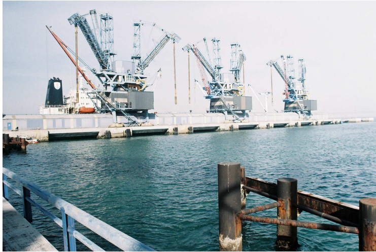
Fig. 1 View of the jetty
